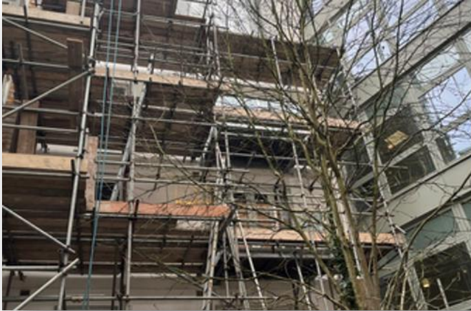
Photo showing Phase 2 North Elevation scaffolding installation works progressing
