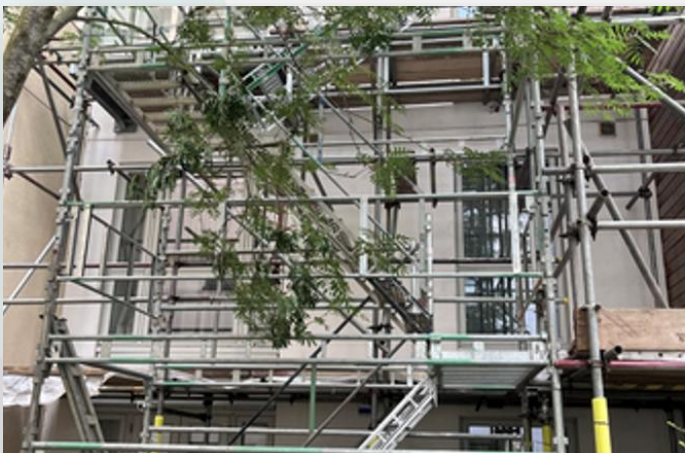
A photo showing Phase 2 North Elevation - HAKI staircase installation works commenced and progressing
