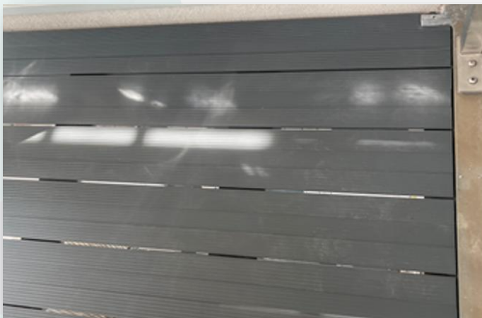
Phase 1 South Elevation
