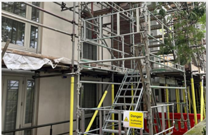
A photo showing Phase 2 North Elevation - HAKI staircase installation works commenced and progressing
