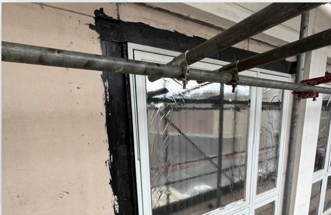
A photo showing Phase 1 South Elevation - New Obex sealing membrane installation
